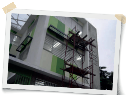
Construction of the Republic of Chile School in Haiti.
